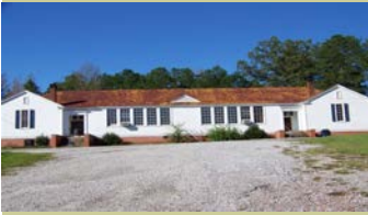
Woodworking Education Center 10544 Hwy 17, Maylene, AL 35114
